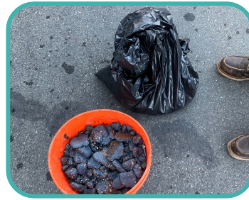
Pool plaster removed from the sewer.
